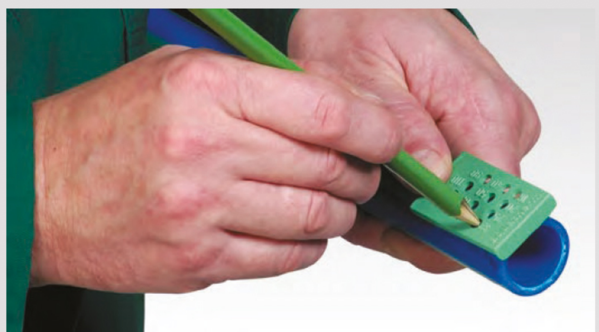
Marking of the welding depth
