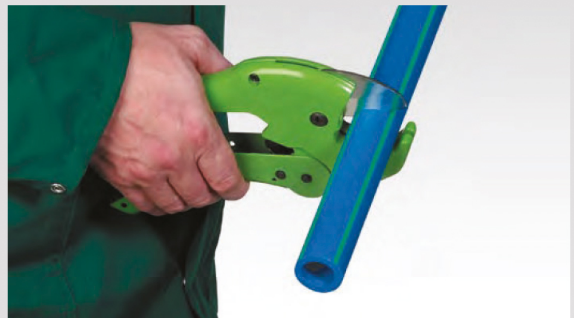
Cutting of the pipe
